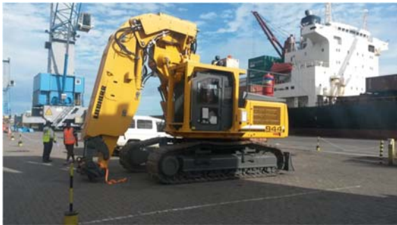
Figure 1 – ACM excavator arriving at port in Mapai
